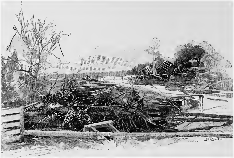
Wreckage on Coosaw Island.
